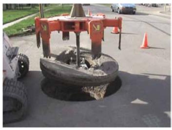
How Does the Mr. Manhole System Work? The Mr. Manhole Six Shooter (shown in the photo) is used to cut and remove the manhole frame and surrounding road material without costly and dangerous physical labor. The repair begins with the Mr. Manhole liner being placed on the manhole cone.
