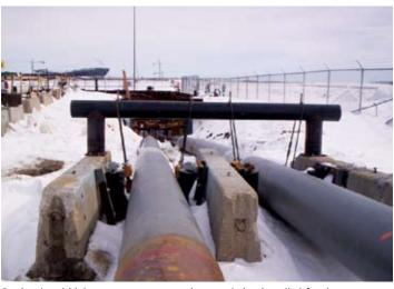
Pre-insulated high temperature water pipes are being installed for the new Midfield Terminal.
