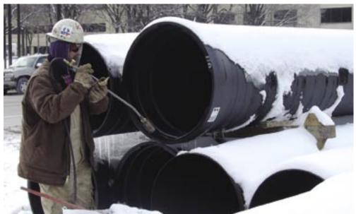
A worker uses a torch to thaw ice that has formed on a section of iron pipe for the chilled water expansion.
