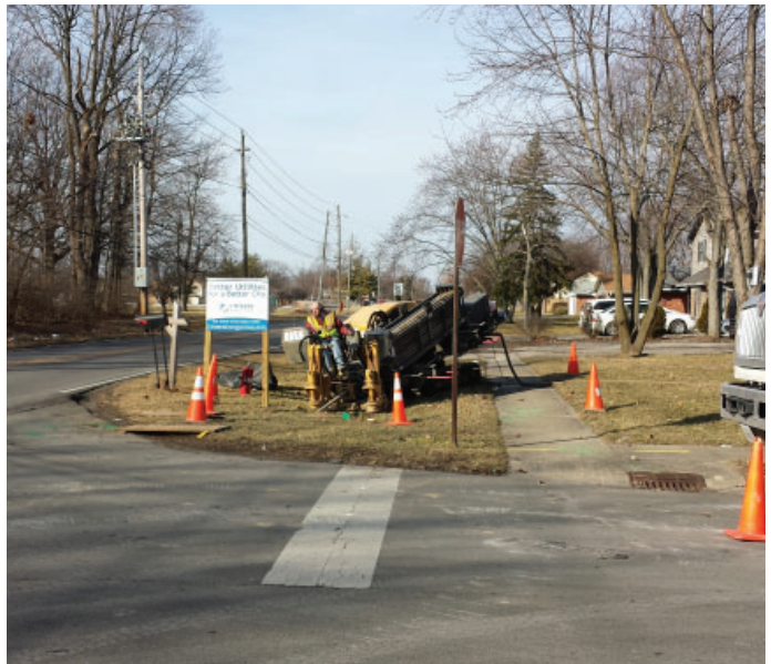
Above: Directional boring machines allow pipe to be installed under streets without disruptive street cutting and excavation.
