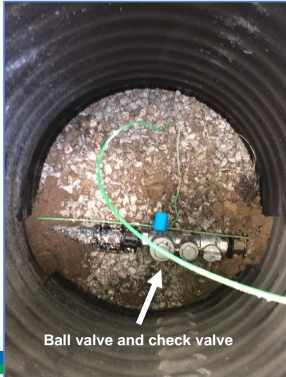
Pictured below: Inside of Service Box/Valve Pit
