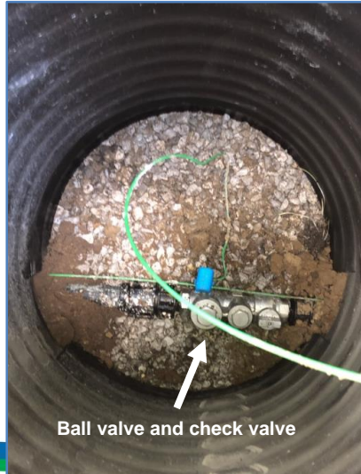
Pictured below: Inside of Service Box/Valve Pit
