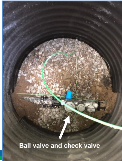
Pictured below: Inside of Service Box/Valve Pit
