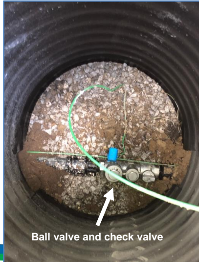
Pictured below: Inside of Service Box/Valve Pit
