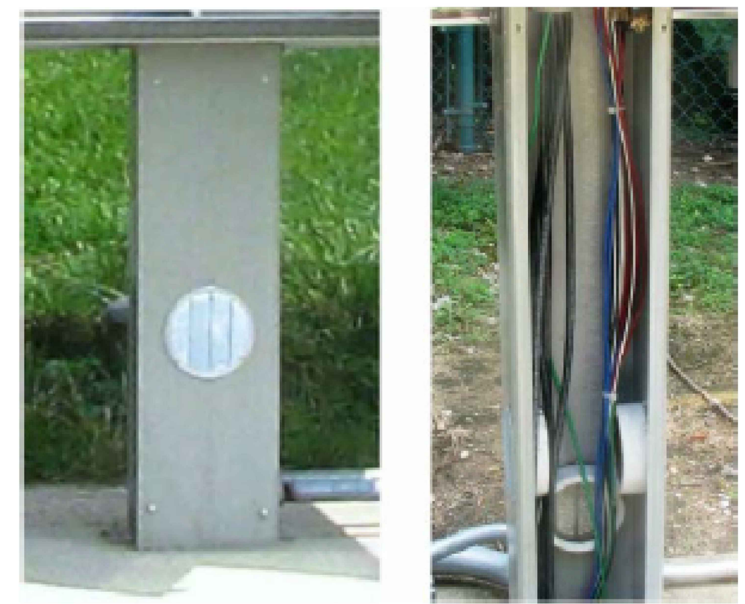
CABLE GUARD DETAIL
