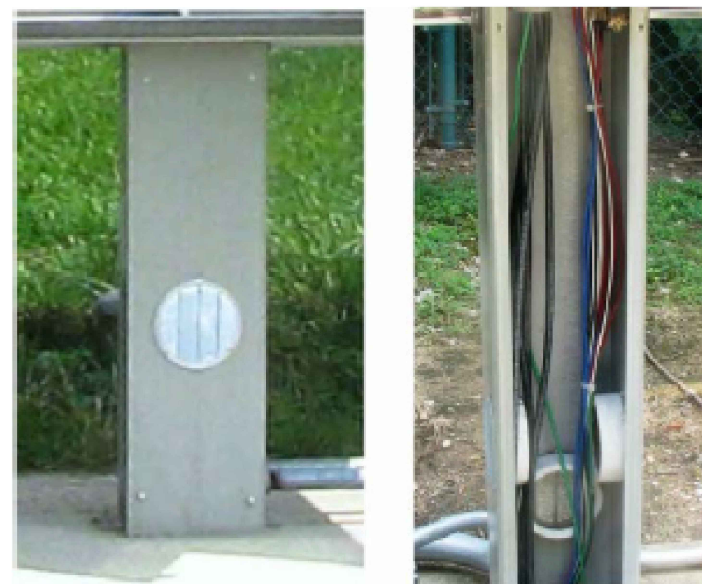
CABLE GUARD DETAIL
