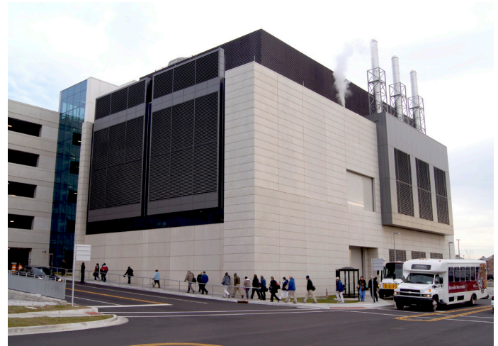
Citizens owns and operates this chiller and steam plant at the Eskenazi Health facility.
