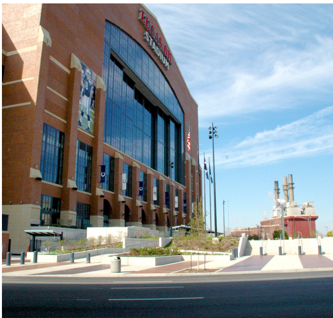
Lucas Oil Stadium depends on efficient steam and chilled water service from Citizens.
