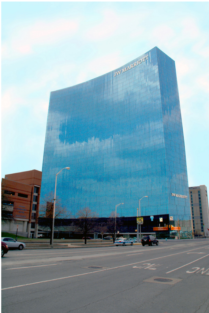
The JW Marriott Indianapolis is one of Citizens latest steam and chilled water customer additions.
