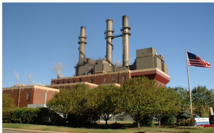
Citizens' Perry K Steam Plant utilizes clean-burning natural gas in its 8 boilers to generate 240°-600°F steam to heat buildings throughout the downtown area.
