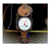
Most water meters are located in a covered meter pit outside of your home. In the case of meters located inside the home, Citizens rules require that they be located in a clean, dry, safe place. All meters, both inside and outside, must be accessible at all times for reading, inspection and removal for
