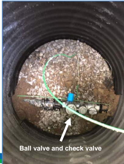
Pictured below: Inside of Service Box/Valve Pit
