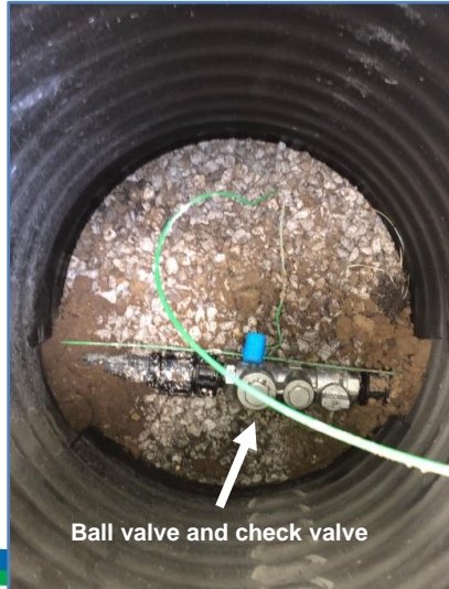
Pictured below: Inside of Service Box/Valve Pit
